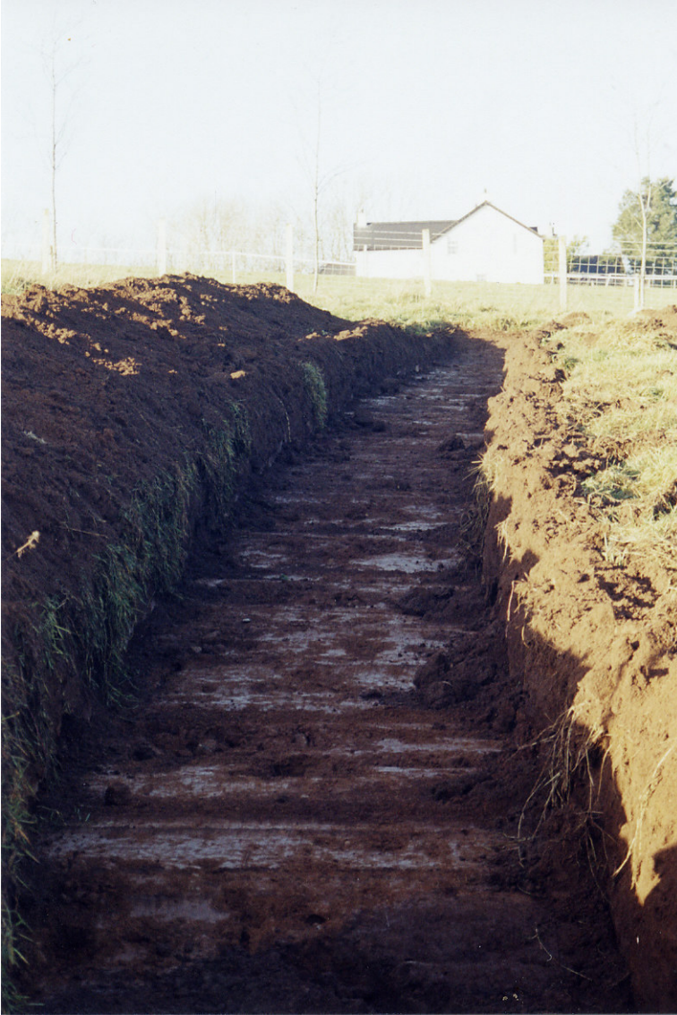
Plate 3: View of Trench 2 from south. Development Site 1 (G/2005/0318/F).
