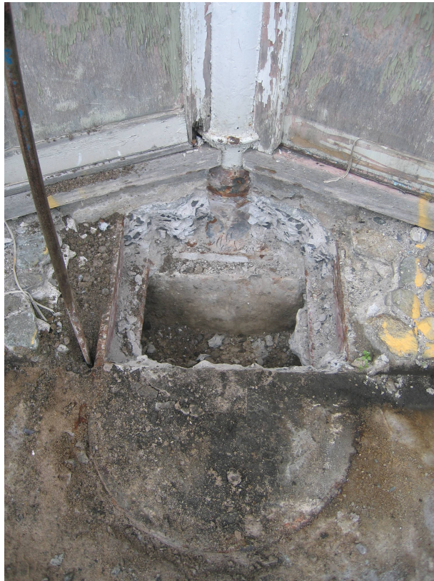
Plate 2: View of Trench A area prior to excavation, showing the cast-iron vehicle kerb (C3), filled with concrete, surrounding the cast-iron pillar (C1) at the southern exterior of the Barrack Coach House.
