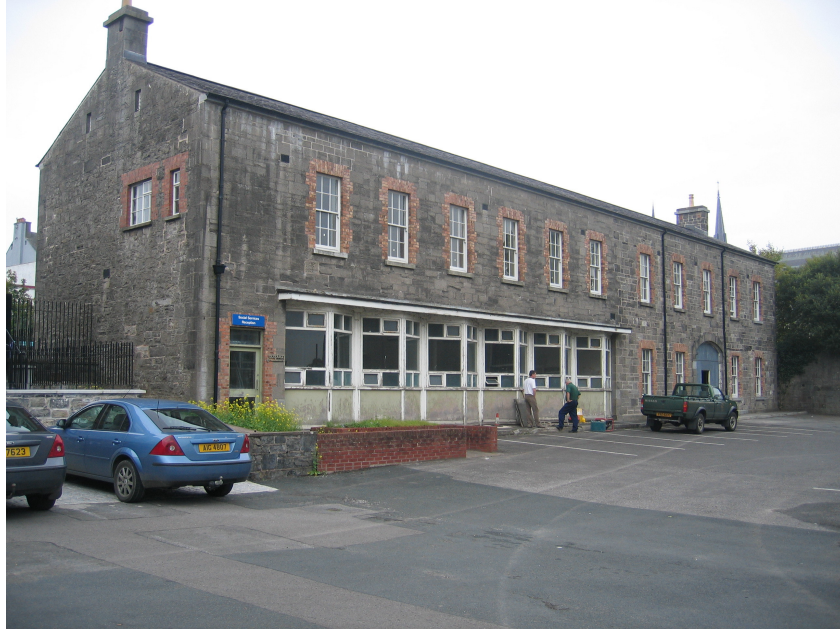
Plate 1: Exterior southern façade of the Barrack Coach House, Enniskillen Castle Barracks
