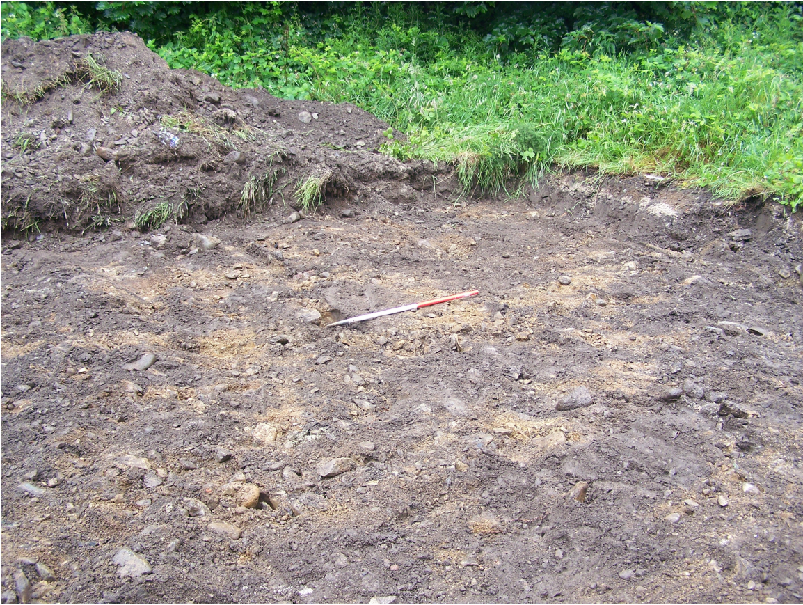
Plate Four: Application site following excavation to the surface of the truncated subsoil (Context No. 102), looking east.
