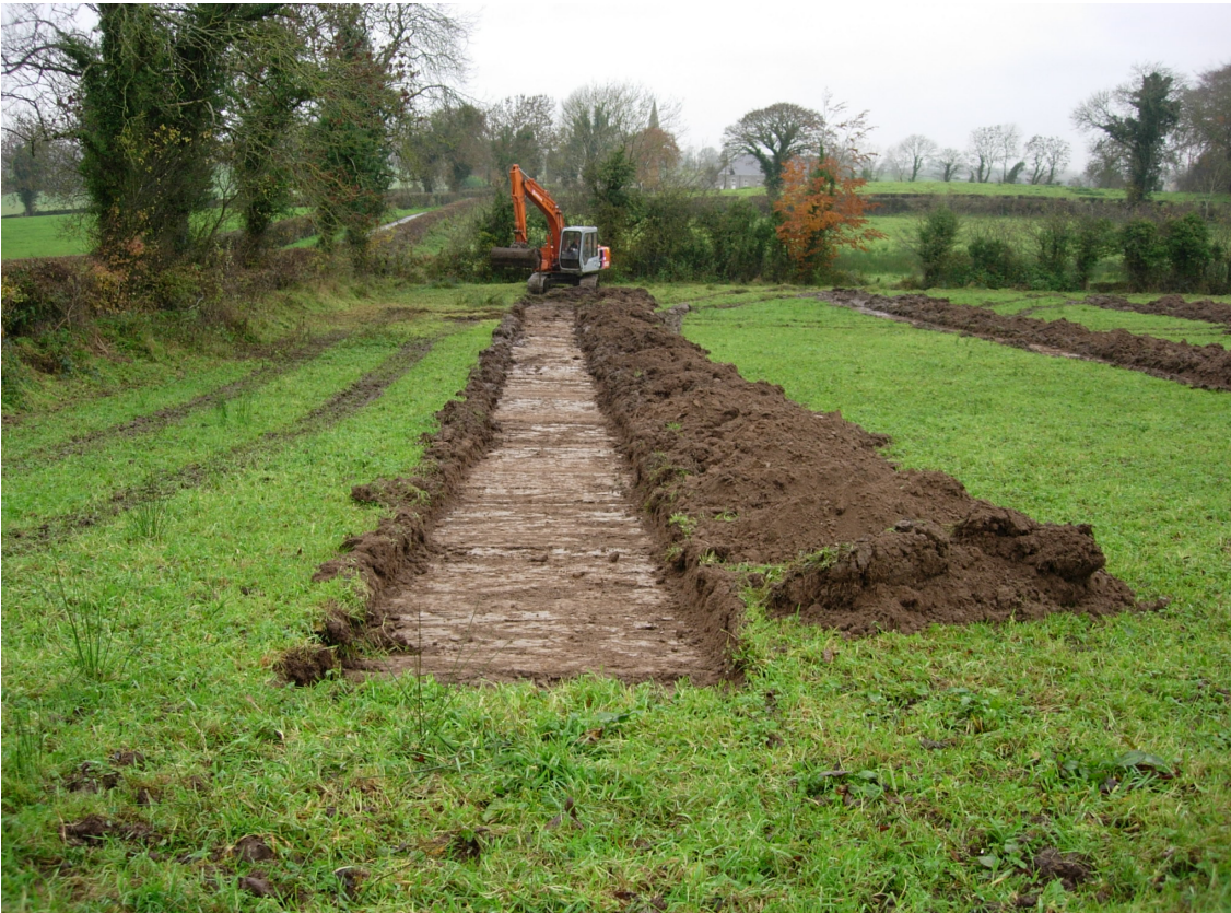
Plate 4: Trench 4, looking north-west.
