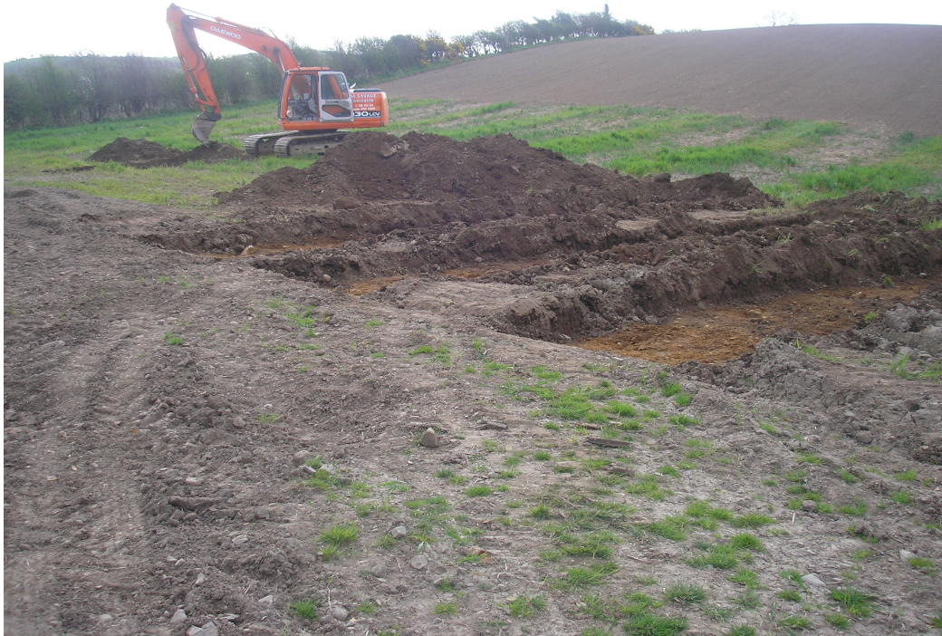
Plate 9: Application site following excavation of the evaluation trenches, looking south-east.
