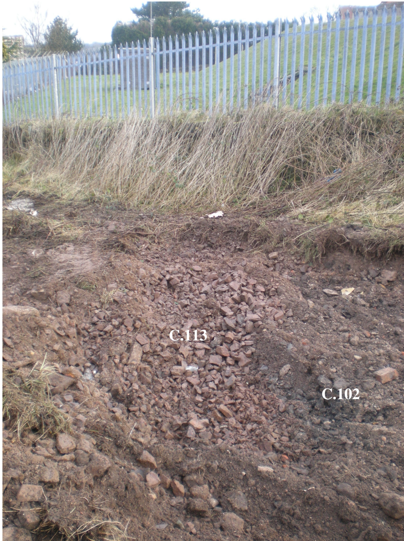
Plate 7 Trench 2: seam of hardcore (C.113) (facing NW).
