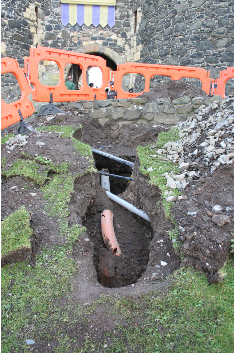
Plate 1: Trench 1 from the north showing existing services.
