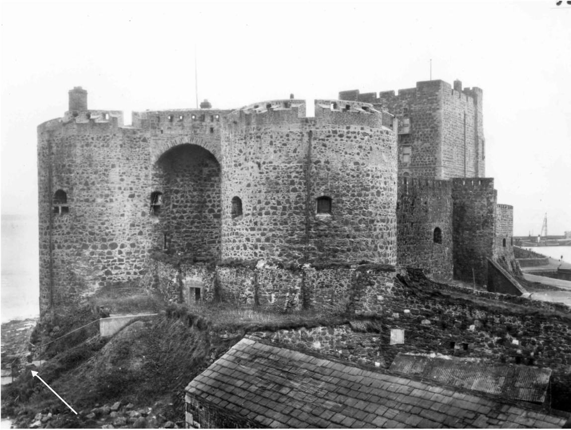
Plate 4: Early 20 th century photograph of Carrickfergus Castle showing possible masonry pier (arrowed) at the base of a staircase with metal handrail.
