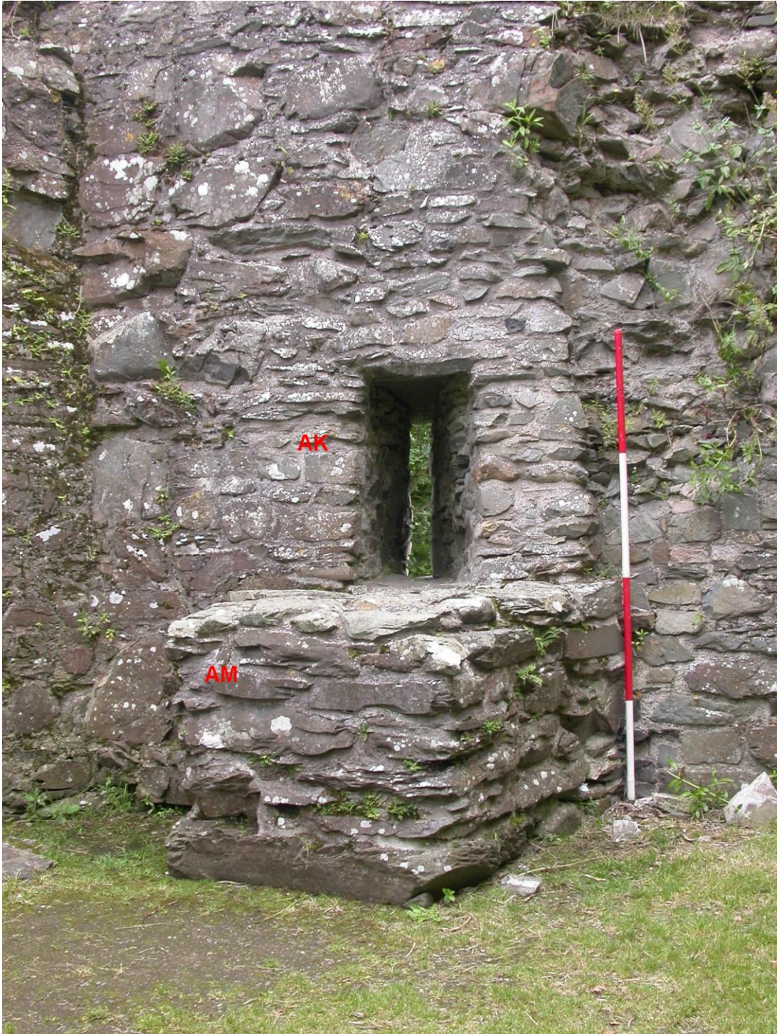
Plate 5: Gun loop (AK), apparently inserted into the lower part of the west wall of the west wing, and associated projecting block of masonry (AM), looking southwest. Scale 2.0 metres.
