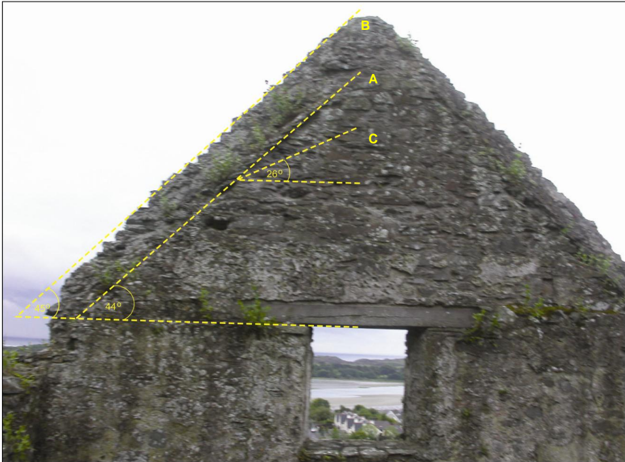
Plate 22: Photographic analysis of the eastern half of the east wing's southern wall. A = 44° angle of the gable to the horizontal (equivalent to the roof's rafter pitch); B = 45° angle of the gabled facade to the horizontal; C = 26° maximum estimated angle of effective pitch of in situ 'slates'.
