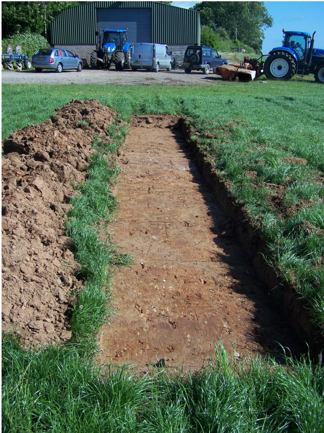
Plate 2: Trench Two following excavation to the surface of the natural subsoil (Context No. 202), looking north.
