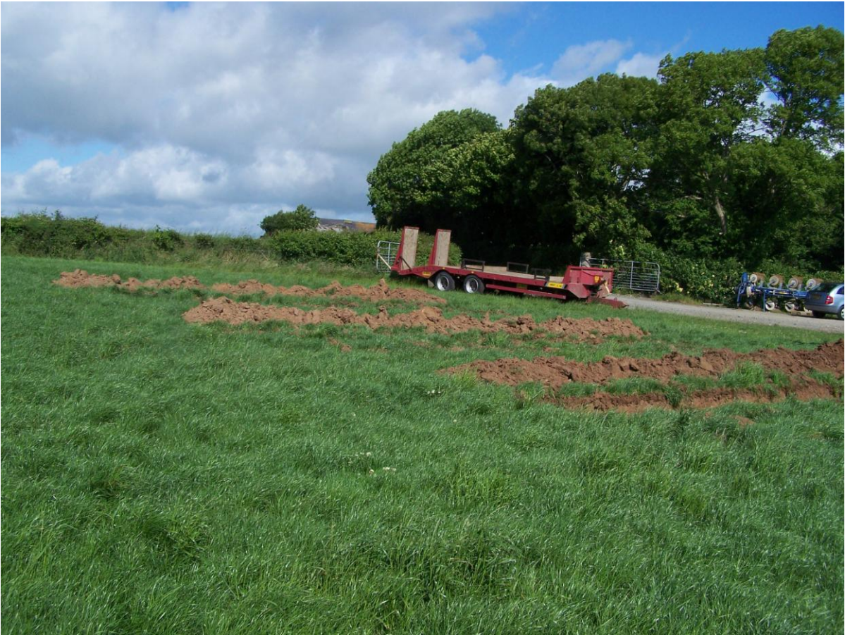
Plate 4: Development site following the excavation of the three evaluative test trenches, looking north-west.
