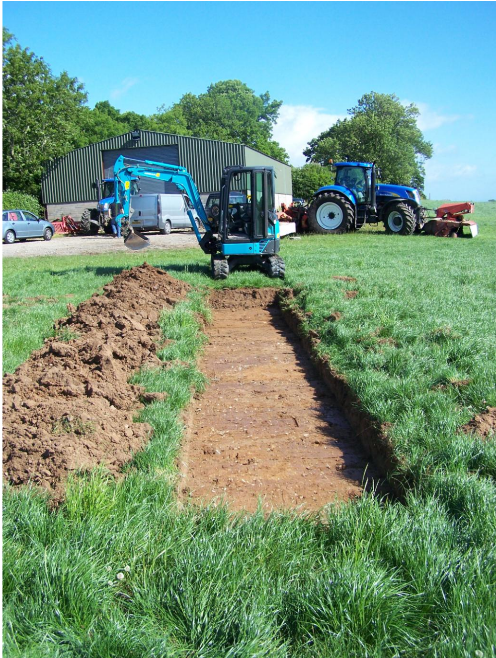
Plate 3: Trench Three following excavation to the surface of the natural subsoil (Context No. 302), looking north.
