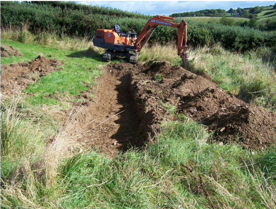
Plate 3: Trench C, post-excavation, looking north-east.
