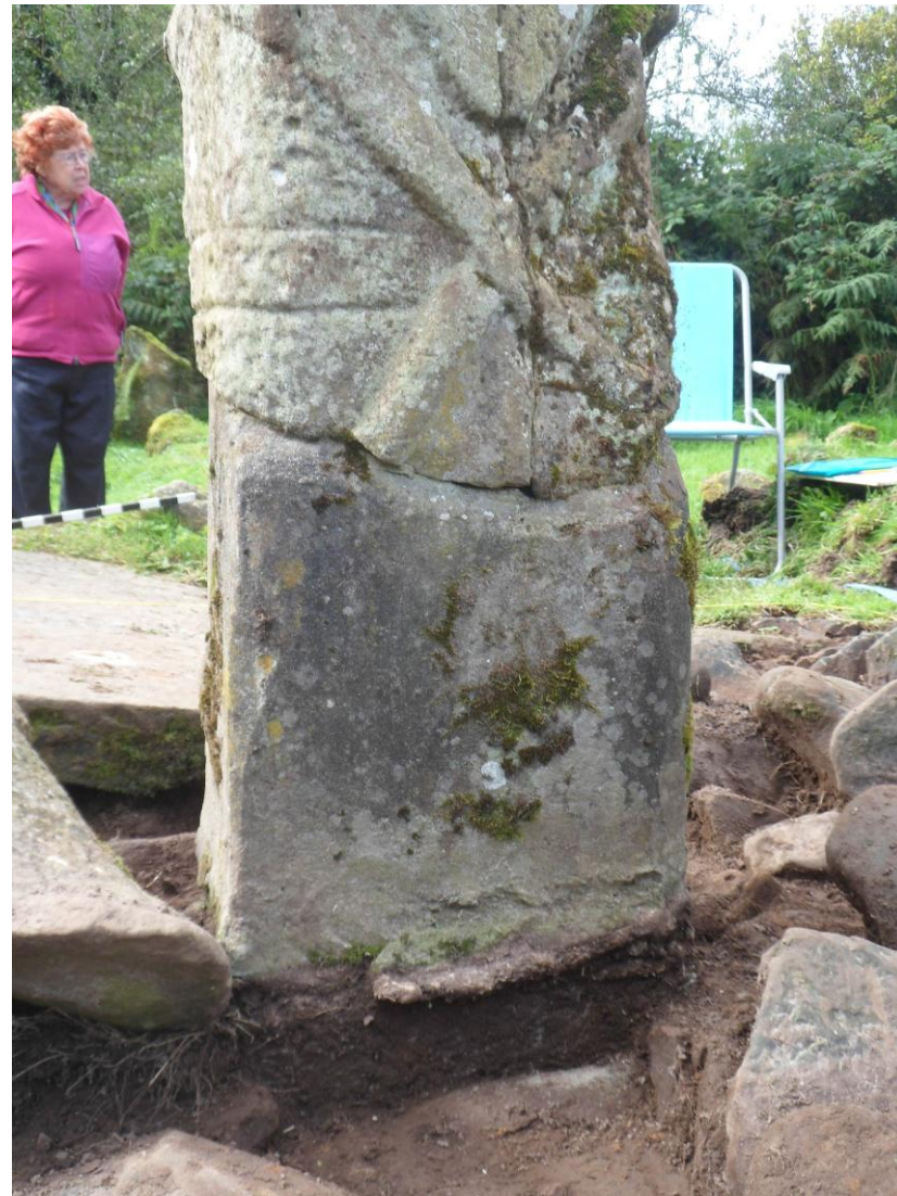
Plate 5 Eastern face of the Boa Island figure showing the two parts of the concrete plinth with the junction marked by the projecting lip of concrete (eastern face).
