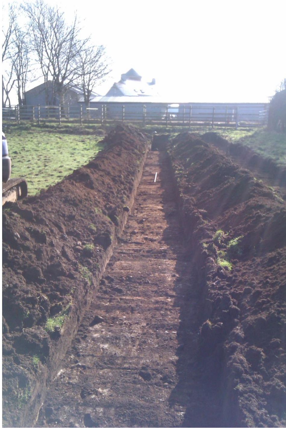
Plate 7: Trench 2, following excavation to subsoil level, looking south-east
