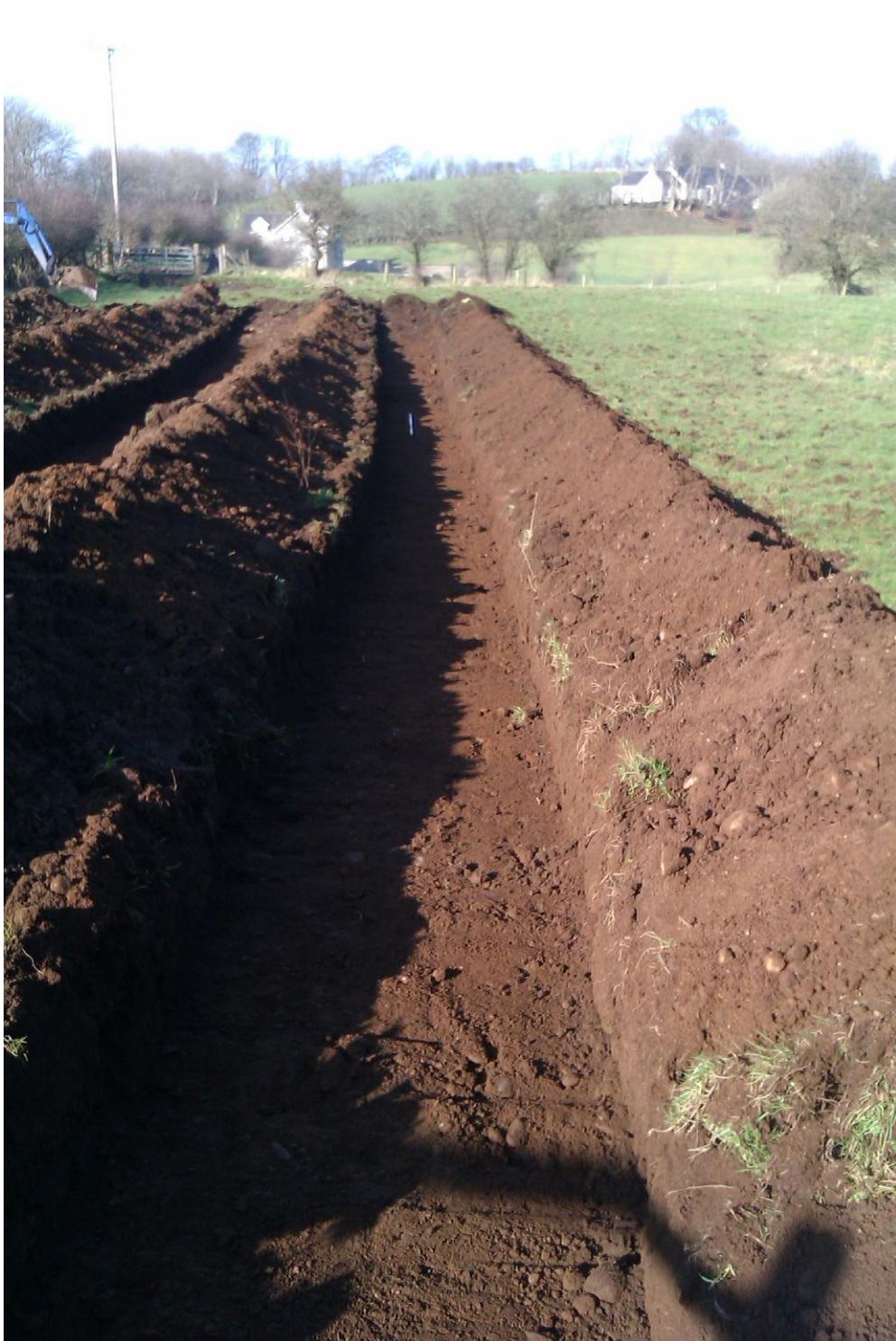
Plate 13: Trench 4 following excavation to subsoil, looking north-west
