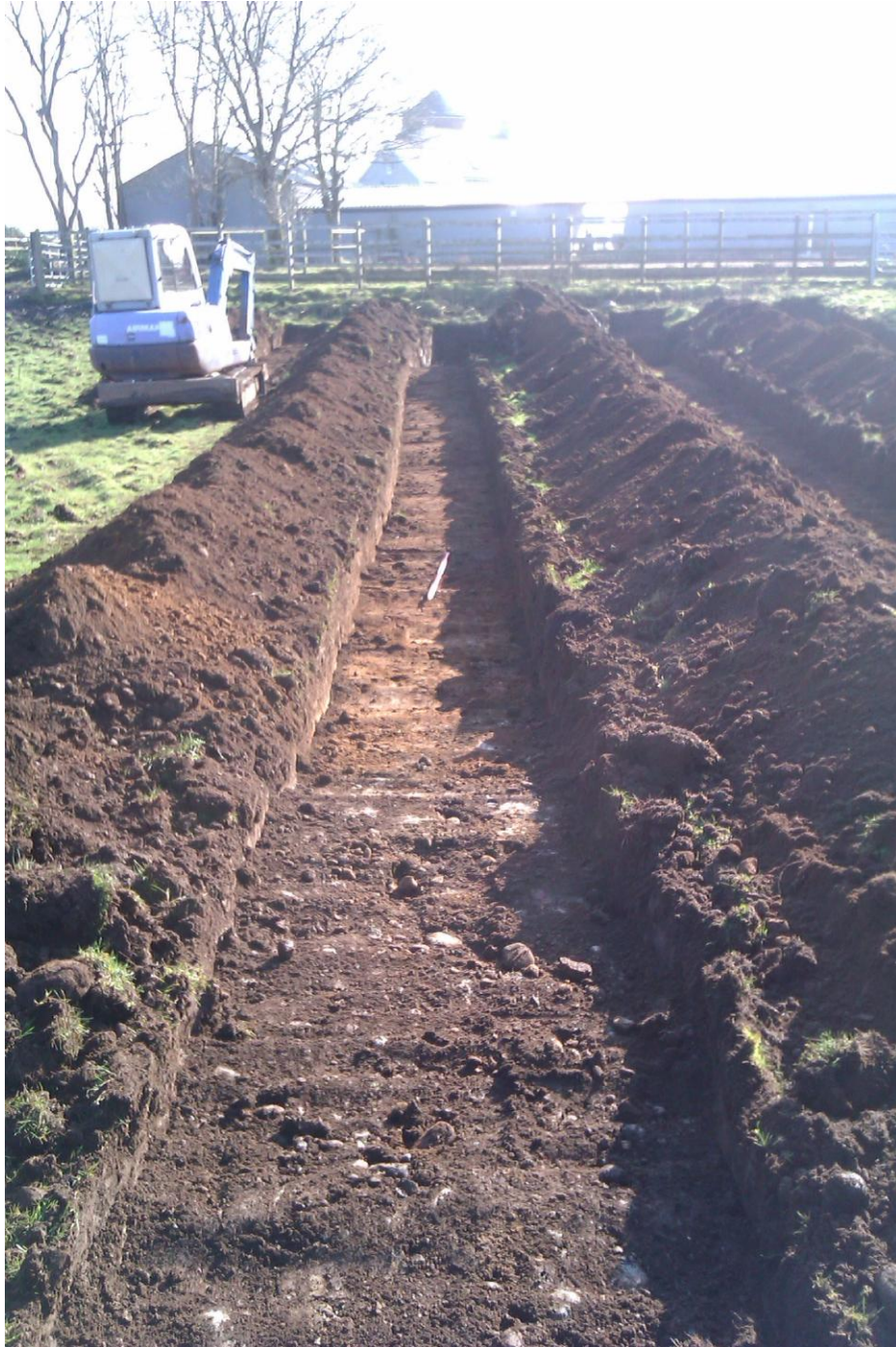
Plate 10: Trench 3 following excavation to subsoil level, looking south-east
