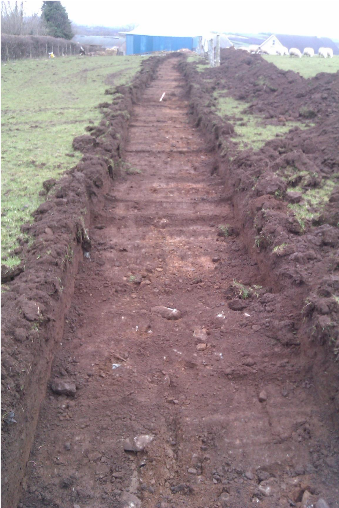
Plate 7: Trench 1 following excavation to subsoil-level, looking west
