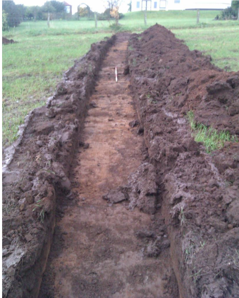
Plate 12: Trench 4, following excavation to subsoil level, looking south
