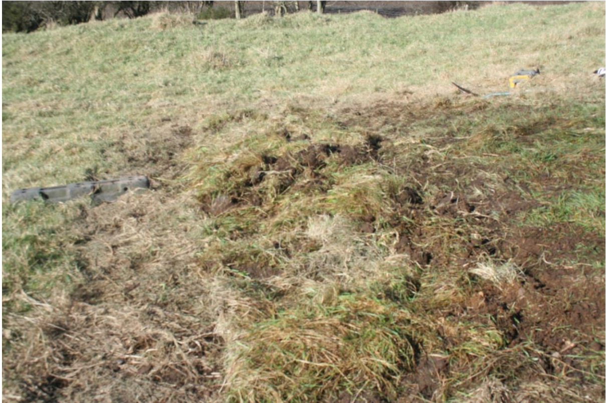
Photo 6: Trench 2 after backfilling
