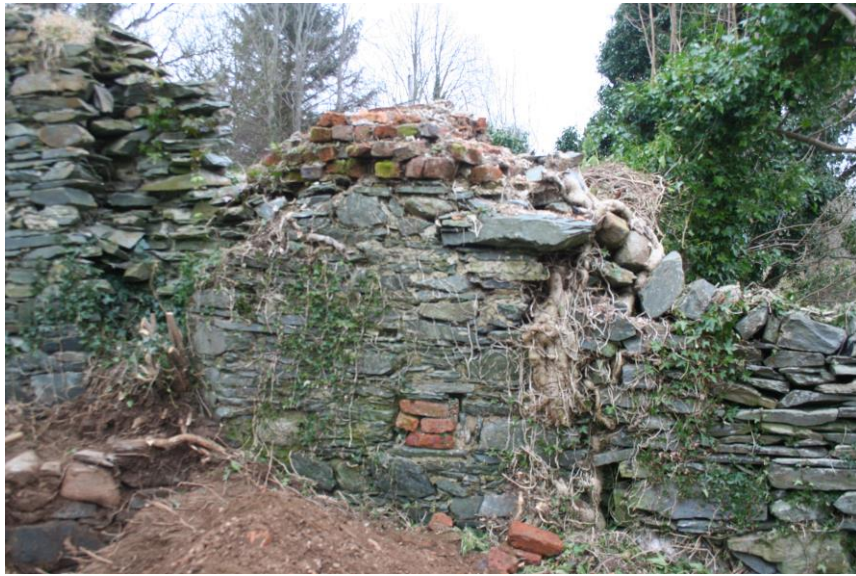
Photo 1: Section of curving masonry from south, showing brick blocked gunloop
