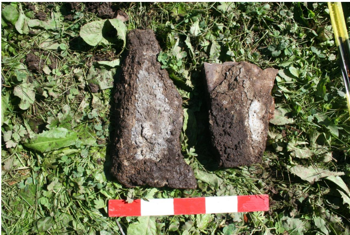
Plate 11: Broken concrete slab from C208
