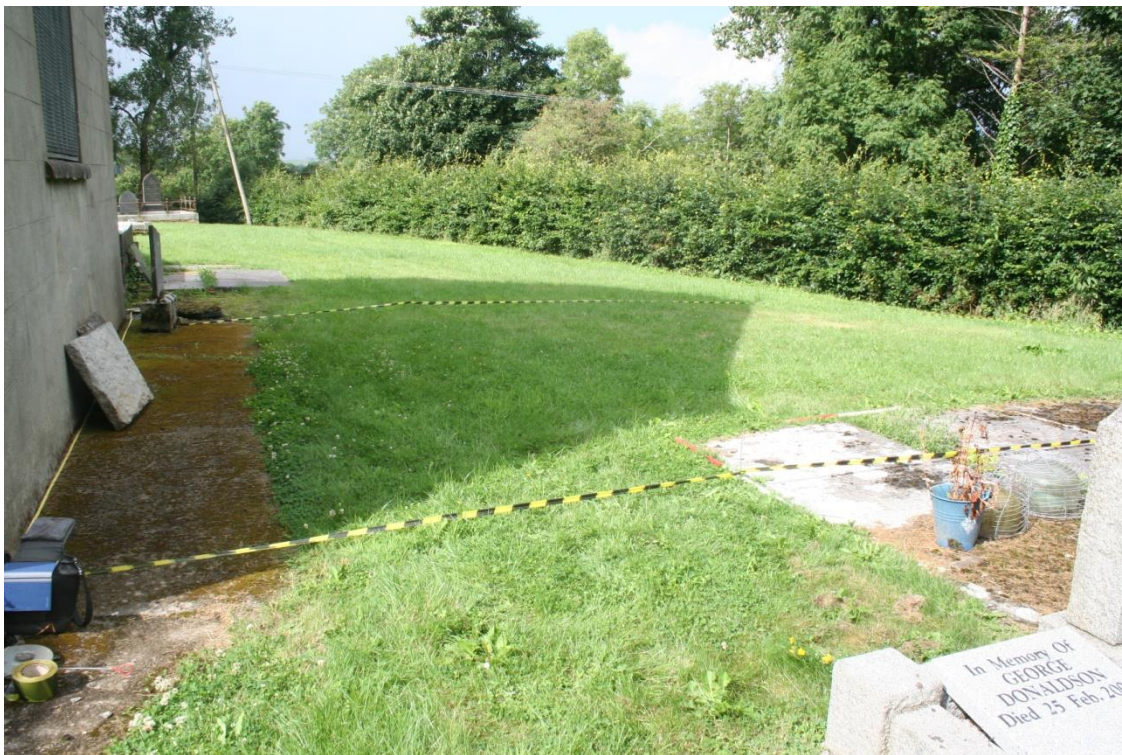
Plate 2: Development area (marked out with hazard tape) showing concrete around base of church, looking West
