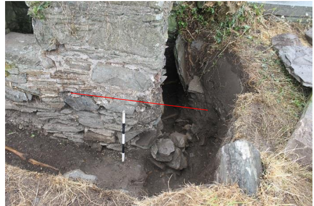
Figure 25 – The eastern end has been tidied, faced and repointed above ground and the below ground portion has remained untouched by the conservation work. It is apparent from the below ground portion of the wall that it would have originally extended further eastwards. The red line indicates the present ground level (Left – looking east-north-east. Right – looking north).
