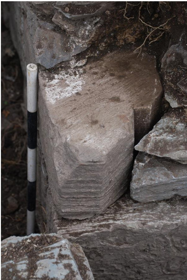
Figure 26 – Dressed stone fragment at the south-west corner, reused in the construction of the 'mortuary house'.
