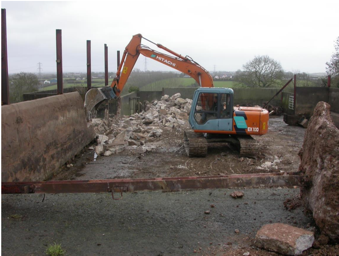
Figure Two: Demolition of the barn in progress, looking east (12.1.11).
