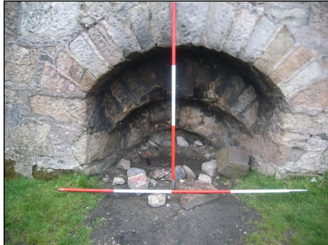
Figure 12: Draw-hole at the Lime Kiln, Murlough Bay
