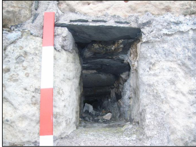
Figure 15: Larger vent at the Lime Kiln, Murlough Bay
