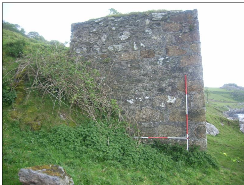
Figure 10: South-facing elevation of the Lime Kiln
