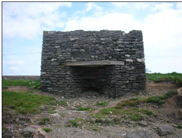
Figure 19: Lime kiln at Hook Peninsula, County Wexford
