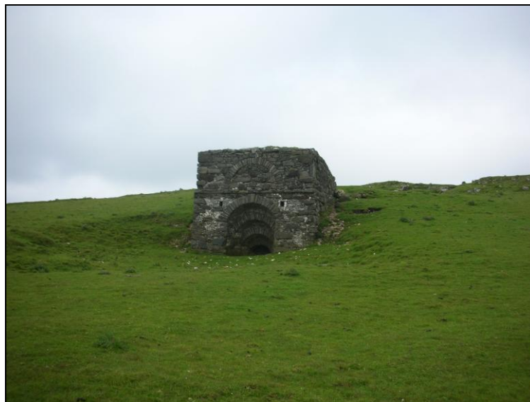
Figure 6: Lime Kiln in the townland of Bighouse
