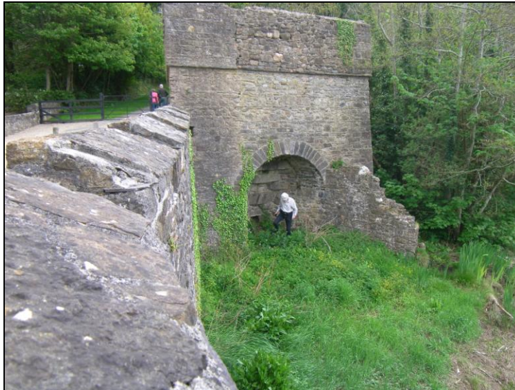
Figure 20: Lime kiln in the grounds of Tintern Abbey, County Wexford
