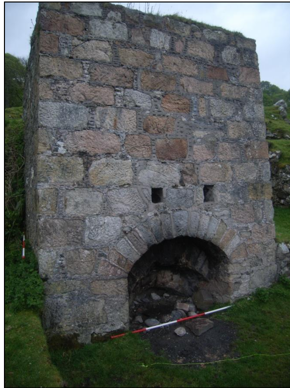
Figure 2: East-facing elevation of the Lime Kiln, Murlough Bay
