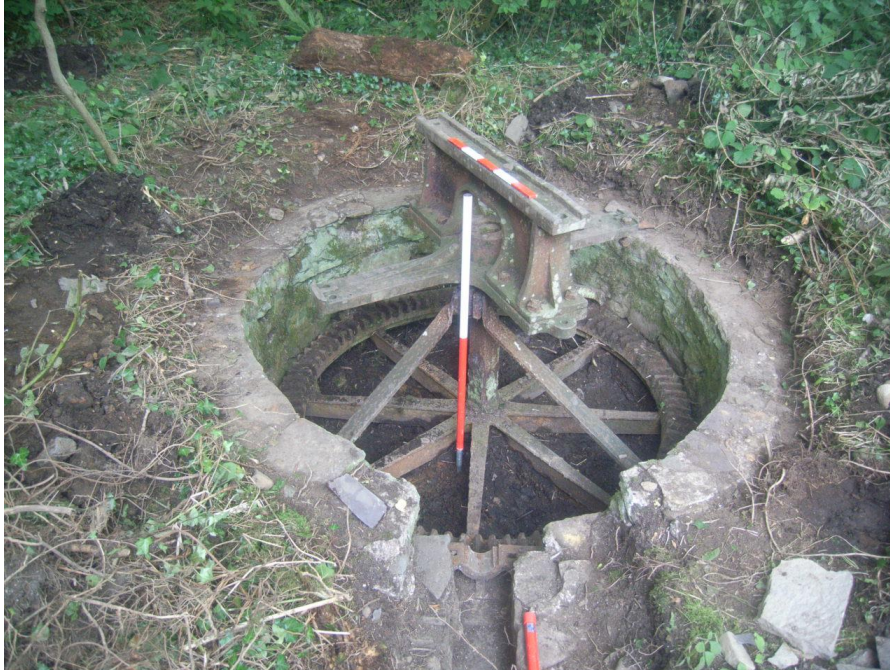
Figure 09: Cog wheel, supporting struts and rotating arms [scales 1m vertical, 0.5m horizontal]
