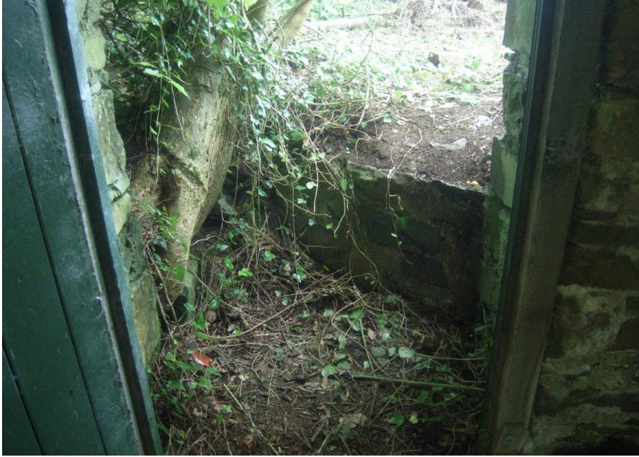
Figure 11: Revetment to horse walk at east of Structure A, looking east
