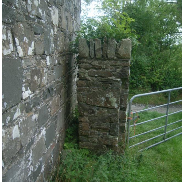
Figure 15: Gate post, looking south
