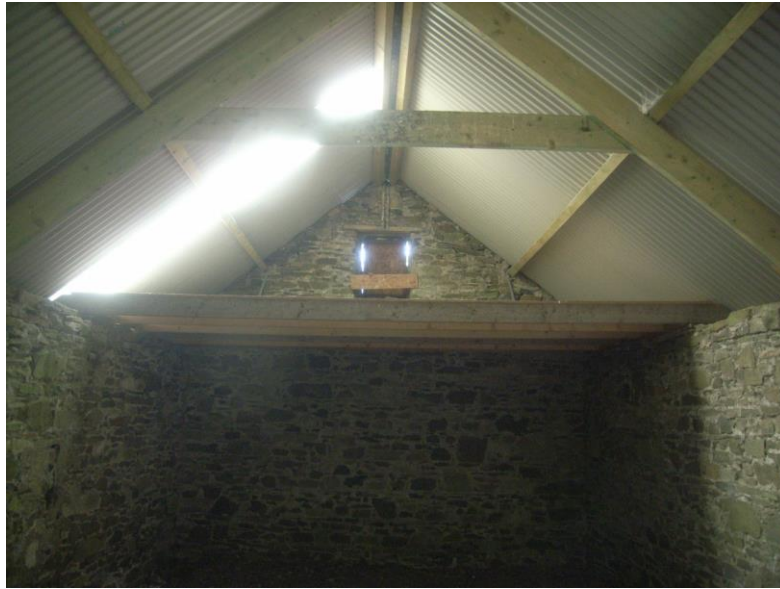
Figure 10: Structure A, with mezzanine and gable window, looking south
