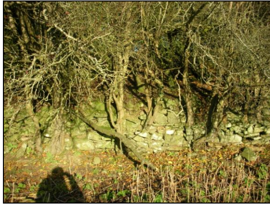
Illustration 3: Stone revetment around external face of bank
