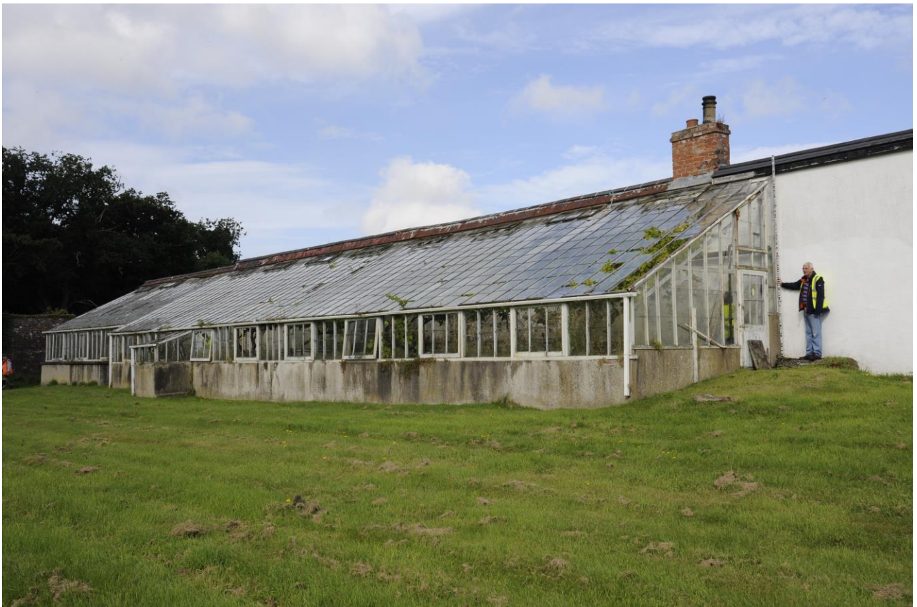
Figure 16. View of Greenhouse from Walled Garden, looking NW
